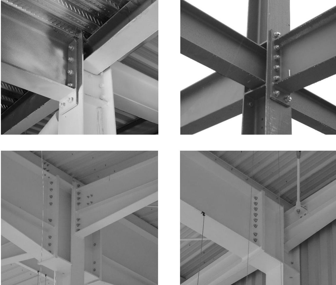
Figure 1.1: Examples of end-plate bolted joints.
