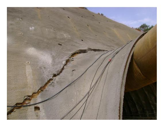
Fig. 7. Fissure developed above the North portal lining.
