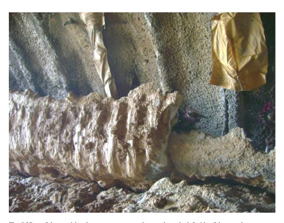
Fig. 8 View of the provisional mortar gutter rotated upwards on the left side of the tunnel
