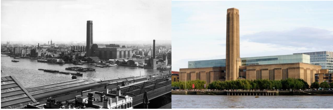
56 e 57. Central elétrica Bankside Power Station, agora Tate Modern, Londres
