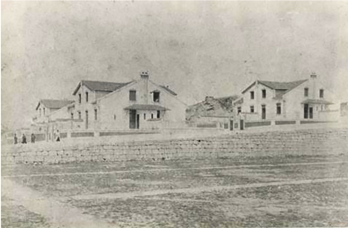
16 Comércio do Porto workers’ houses, designed by José Marques da Silva, Porto, 1905, FIMS (FIMS/MSMS/Foto0119).
