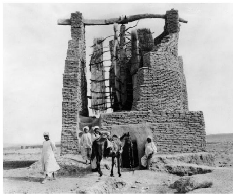
a. Vertical-axis windmill for milling grains, Afghanistan
