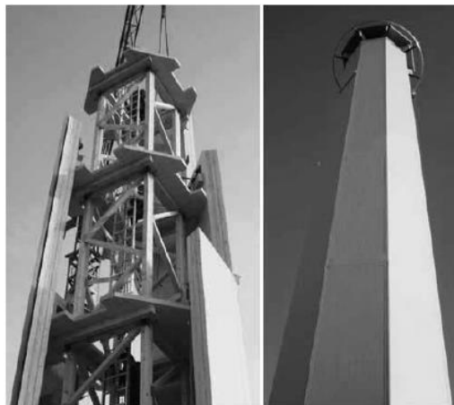
Figure 3.8: Timber wind tower (Engström et al., 2010)
