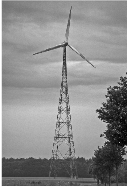
Figure 2.5 - Lattice tower of a Vestas V80 wind turbine (Hau, 2013)
