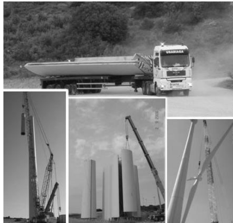
Figure 3.5: Modular concrete INNEO tower (INNEO Torres, 2008)
