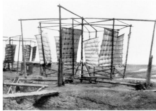
b. Ancient chinese windwheel for pumping water and draining rice fields
