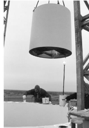
b. Erection of a prefabricated prestressed-concrete tower for an E-66
