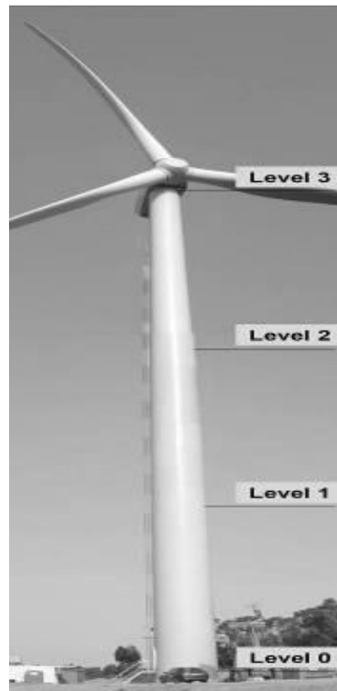
Figure 2.8 - Instrumented tower in Marvila, Portugal
