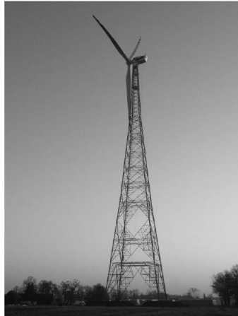
Figure 3.6 - 160m Fuhrländer Wind Turbine Laasow (Almeida, 2015)
