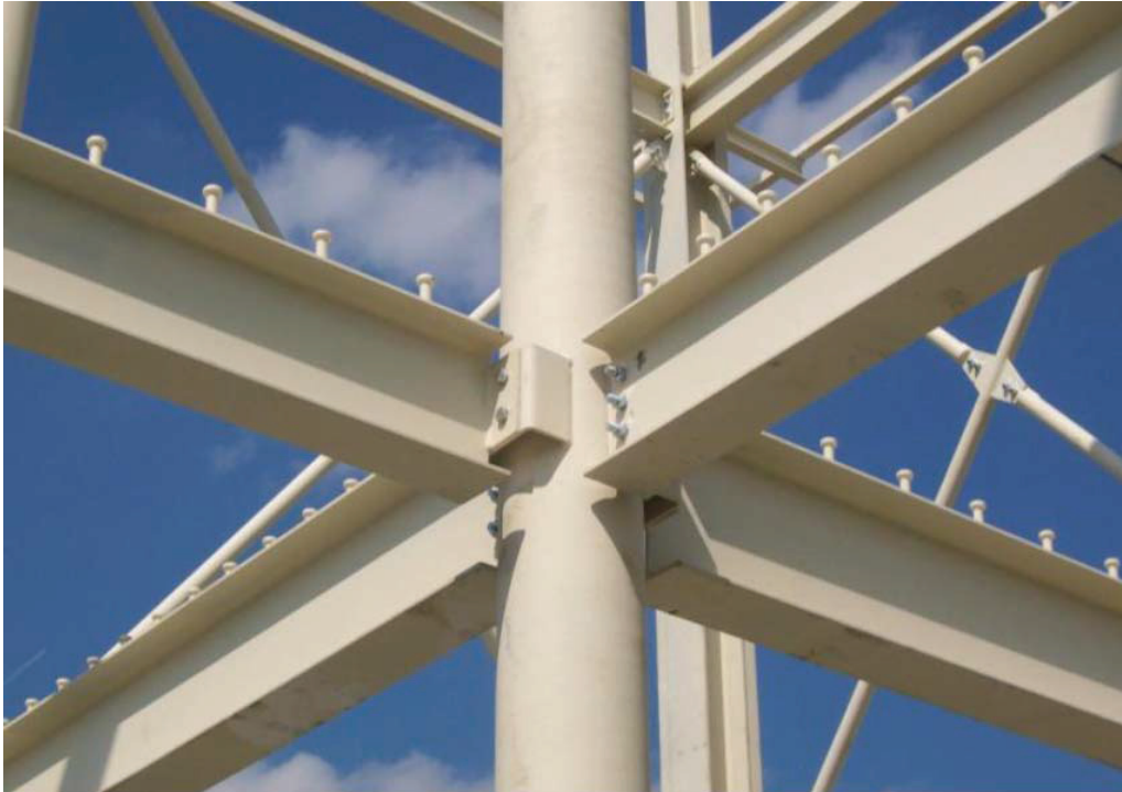
Figure 2.3: Reverse channel and fin plate connections used during the Veseli fire test [43]
