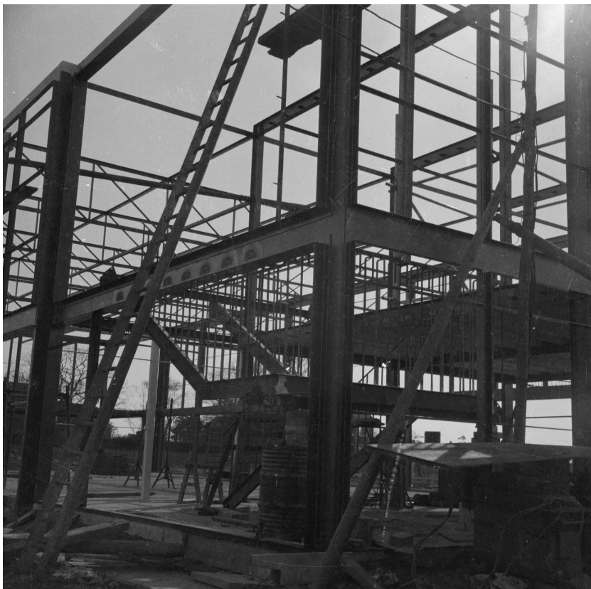
Photograph showing the construction of Hunstanton Secondary Modern School, Norfolk [c 1953]
