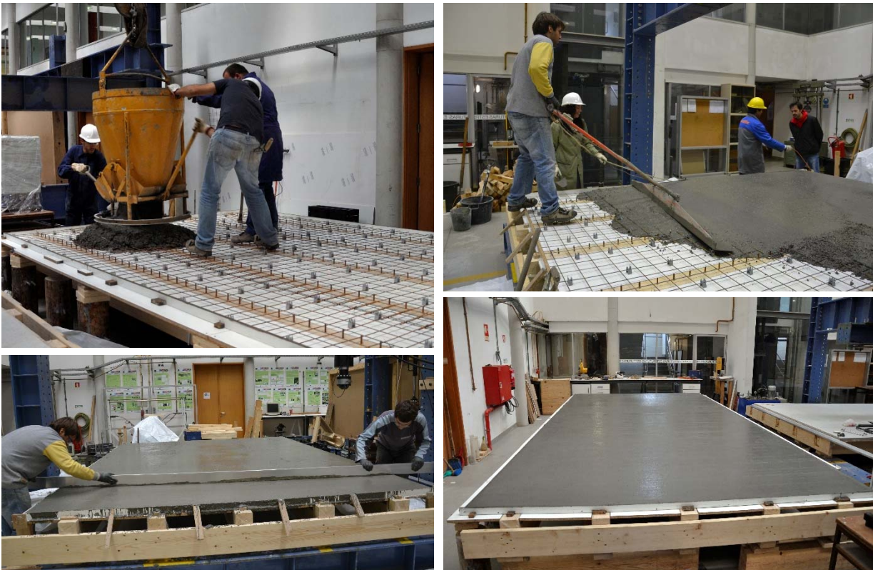
Fig. 4.2 – Casting of the test specimens
