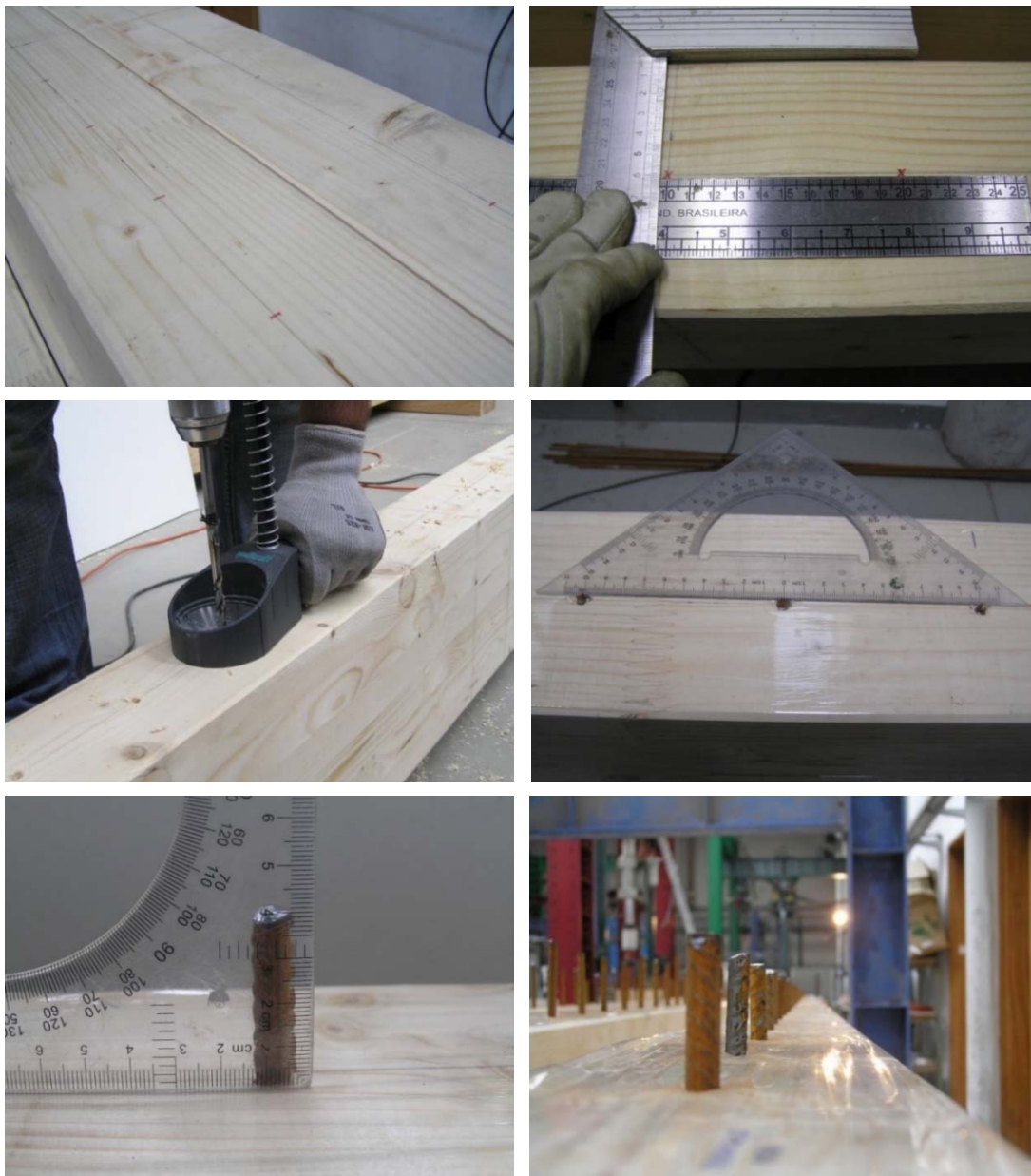
Fig. 4.6 – Placing of the steel rods: marking, drilling and positioning
