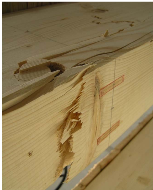
Fig. 4.55 – S3-hc=0.03m B4-GL5 failure
