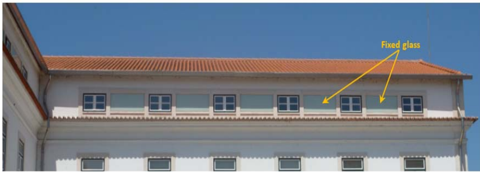
Figure 3.4: Picture of the southeast façade of the 2nd floor.
