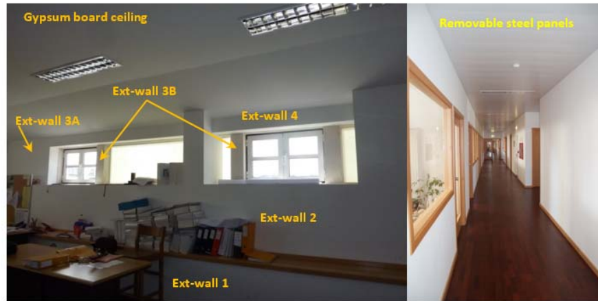
Figure 3.5: Office (left) and corridor (right) pictures of the 2nd floor.
