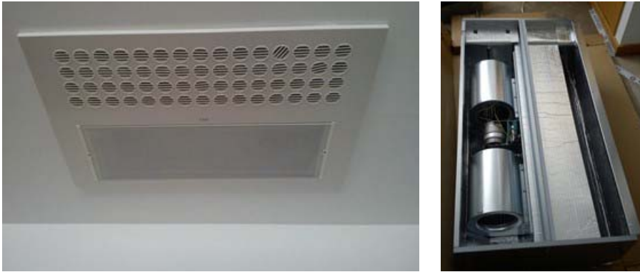
Figure 3.14: Fancoil units.
