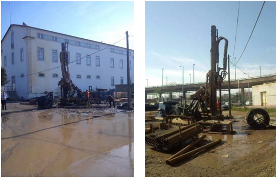
Figure 3.11: Views of the drilling site.
