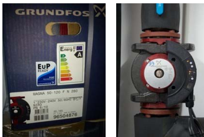
Figure 3.12: Images of the circulation pumps
