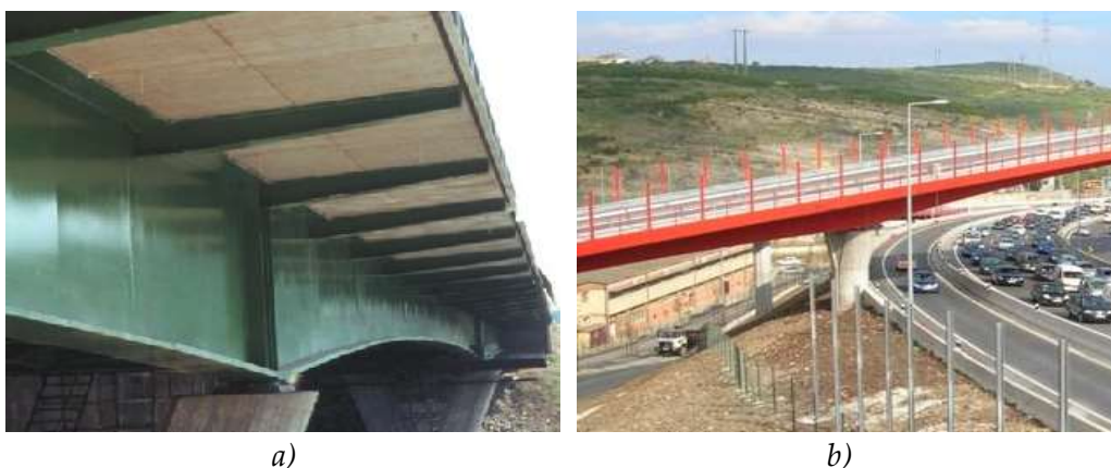
Figure 1.6: a) Bridge over Rio Ave, Portugal and b) Bridge over IC19 in Lisbon, Portugal (courtesy of Professor António Reis)
