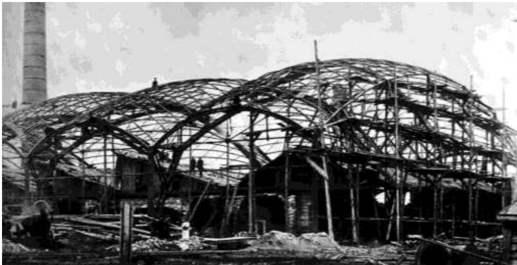
Figure 1.1: Diagrid Shell by Vladimir Shukhov during construction, Russia (unknown author, 1897)
