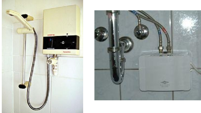
Figure 4.1: Examples of POU tankless water heater used in Britain and Germany.
