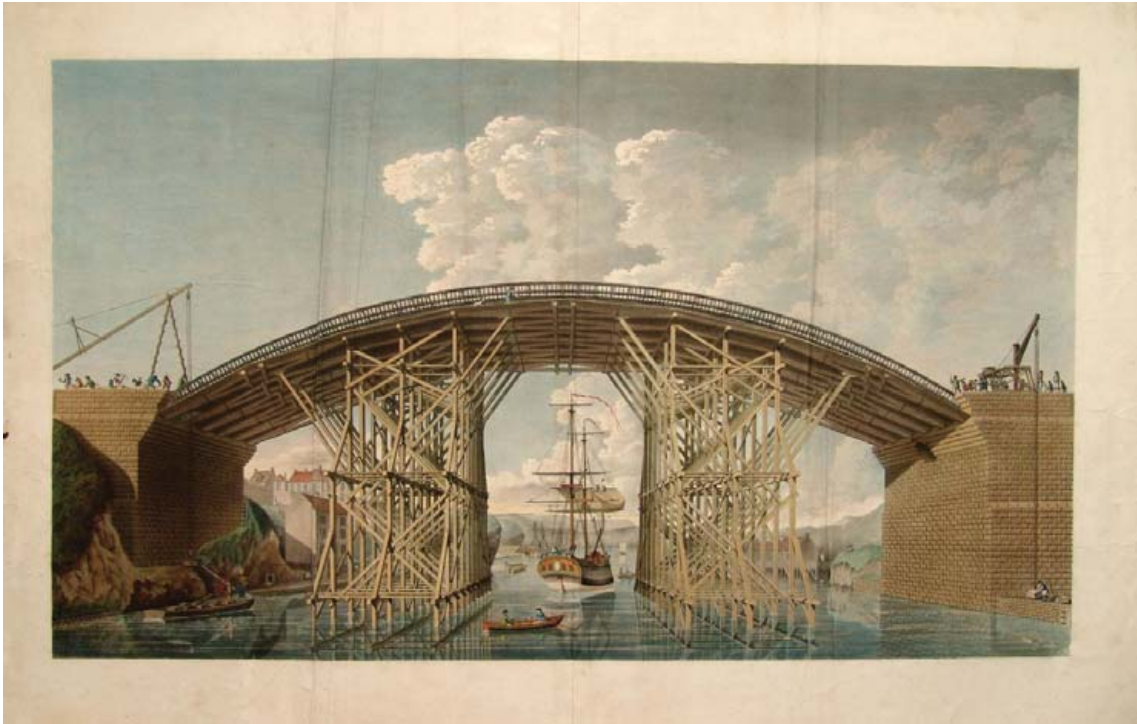
Fig. 157, [CLARKE, Robert, To Rowland Burdon Esqr M.P. by Whom this Excellent piece of Mechanism was invented & under whose Patronage it has been carried into Execution This East view of the Cast Iron Bridge over the River Wear at Sunderland in the County of Durham, previous to the Centre being taken down, Is respectfully dedicated by His humble Servant Robert Clarke, Rpb. Clarke Del. J. Raffield sculpt., Publish'd Octr. 1st, 1796. by J. & J. Taylor at the Architectural Library High Holborn, 1796 ], Arquivo BPMP, C-M&A, 20(30).
