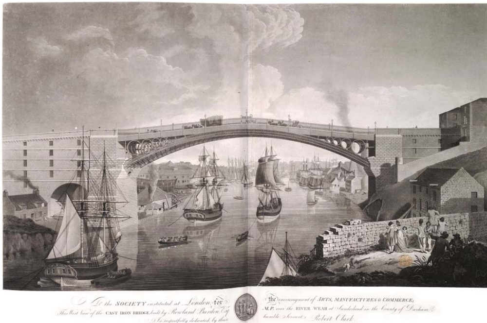
Fig. 158, CLARKE, Robert, To the Society instituted at London, for the Encouragement of Arts, Manufactures and Commerce; This West View of the Cast Iron Bridge built by Rowland Burdon, Esq.r M.P. over the River Wear at Sunderland in the County of Durham, Is respectfully dedicated, by their humble Servant, Robert Clark, Rob.t Clarke del. J.Raffike sculp.t. Publish'd Feb.y 1st 1798, by J. & J. Taylor, at the Architectural Library, High Holborn.
