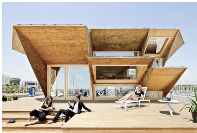
Fig. 21 – Endessa Pavilion – Institute for Advanced Architecture of Catalonia (2011).
