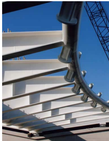
Figure 1.9 Three bridges over the Hoofdvaart Haarlemmermeer, the Netherlands (Steel Construct (no date) [online])
