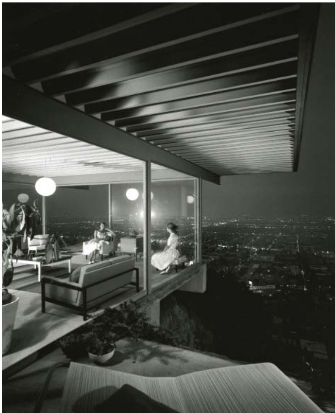
35. Case Study House #22, projectada sobre Los Angeles (Los Angeles, E.U.A., 1960) f. Julius Shulman a. Pierre Koenig
