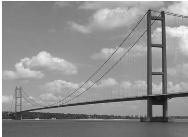
Figura 2.30 – Humber Bridge, com vão central de 1410 m<sup>13</sup>.
