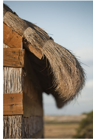
Figura 3.3 - Pormenor de cobertura ( http://www.archdaily.com )
