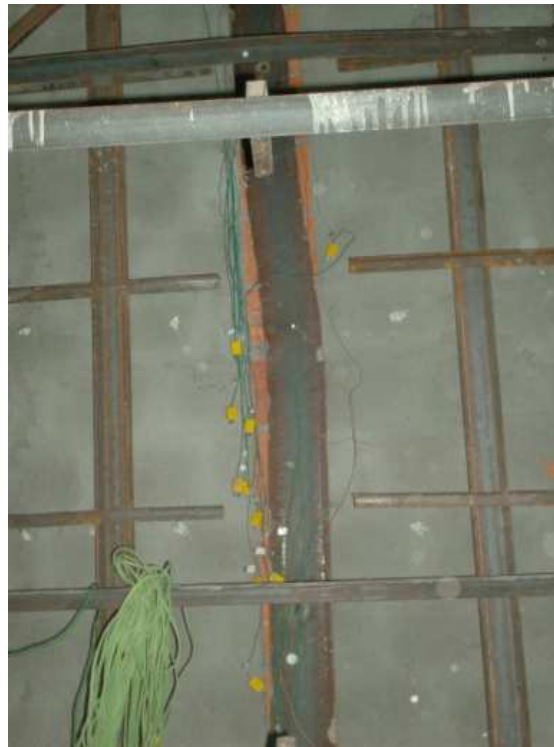
Figure 4.52 - Column E13 after test - web perpendicular to wall – wall thickness 100mm - HEA 160
