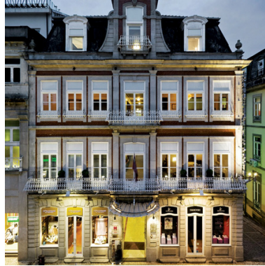
Fig. 40 - Fachada do Grande Hotel do Porto ( http://images.channels.nl/1/images/hotel/max500/111/1116637.jpg )
