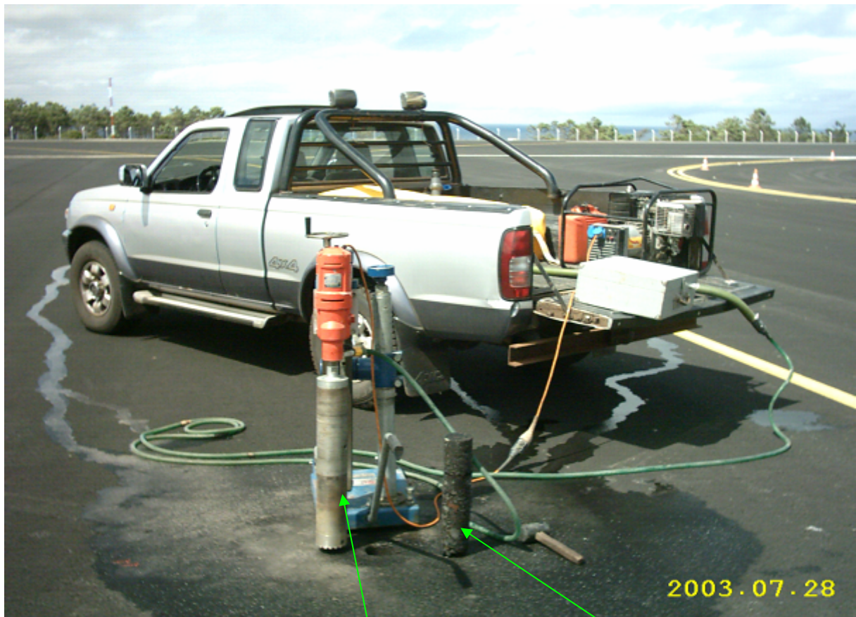
Figure 3.18 – Core drilling equipment and extracted core
