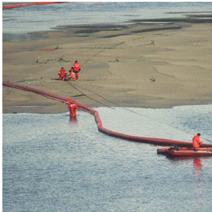
Fig. (2). Surface controlled net for collecting the crude and oil adsorbing elements (November 2002).
