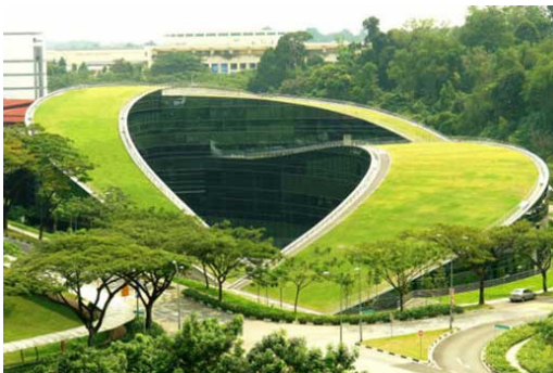
3.17 – California Green Roof Art School, CPG Consultants Pte, Singapura ( http://www.archicentral.com/tag/green-roof/ )
