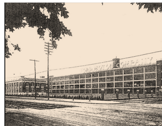
Automobile Assembly Building , Highland Park, Detroit, 1909, Albert Kahn
