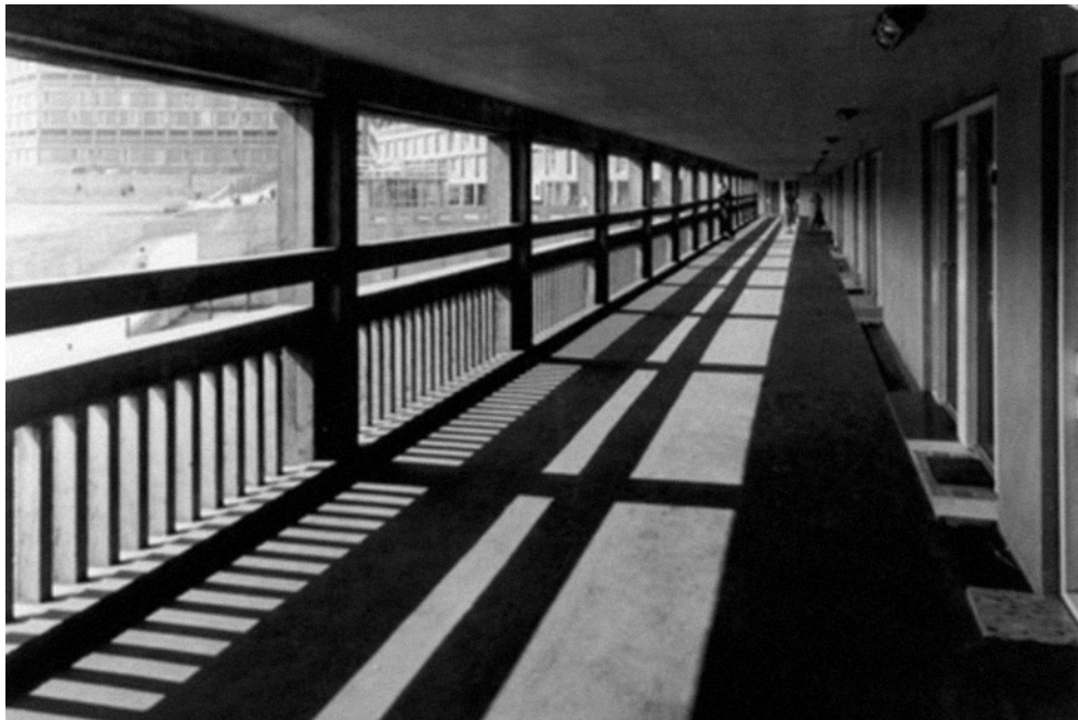
fig.29 Park Hill Flats, galeria de acessos, Alison e Peter Smithson, 1957-61, Sheffield
