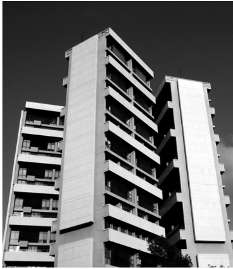
fig.30 Keeling House, Denys Lasdun, 1954-57
