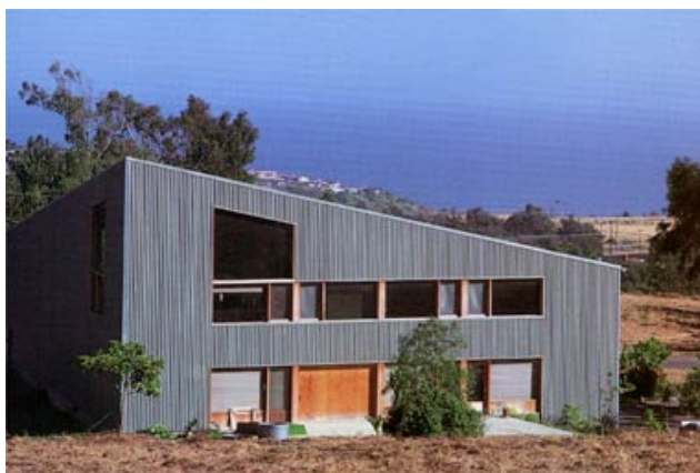
Fig.53-Davis Studio and Residence
