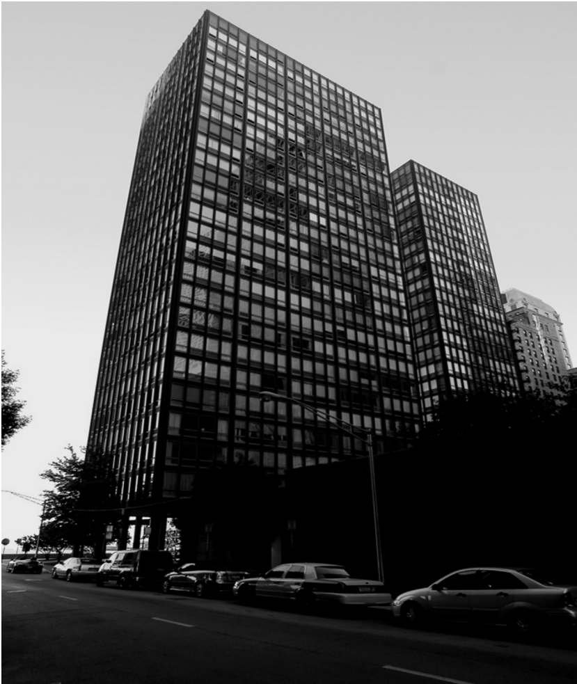
FIG. 9 Apartamentos Lake Shore Drive, Mies van der Rohe, Chicago, 1948-51.
