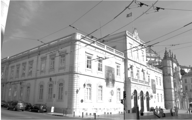
Figure 6 The New City Hall next to the Church of Santa Cruz
