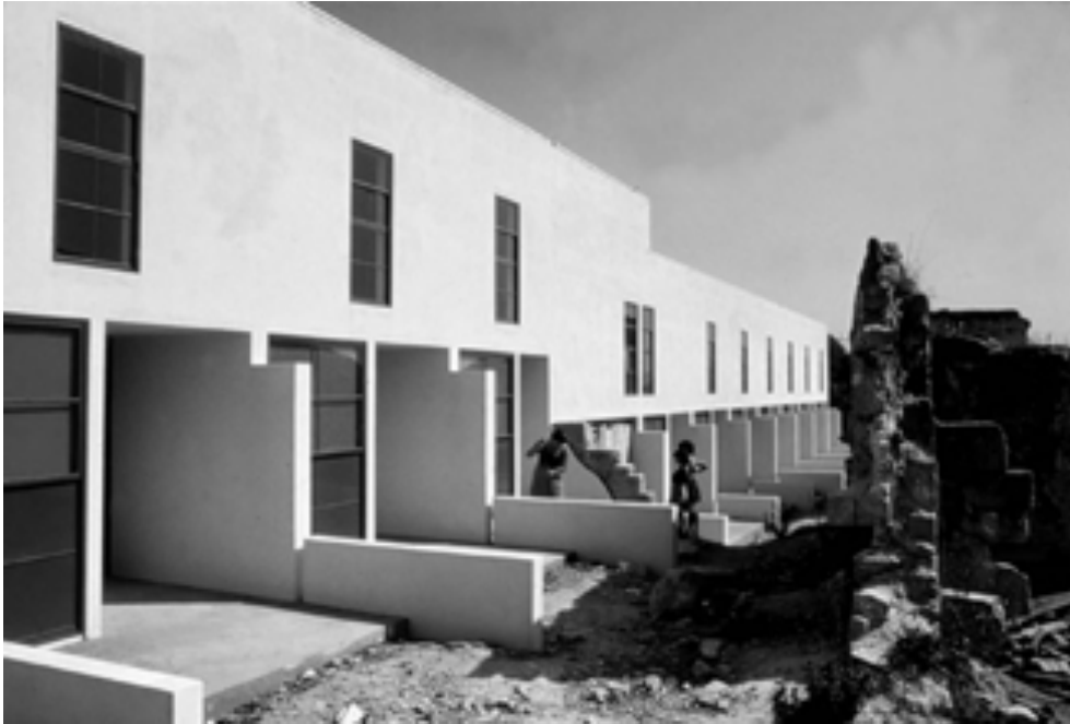
Figure 1. Álvaro Siza. First row houses built in São Vitor. © Credits Alexandre Alves Costa.
