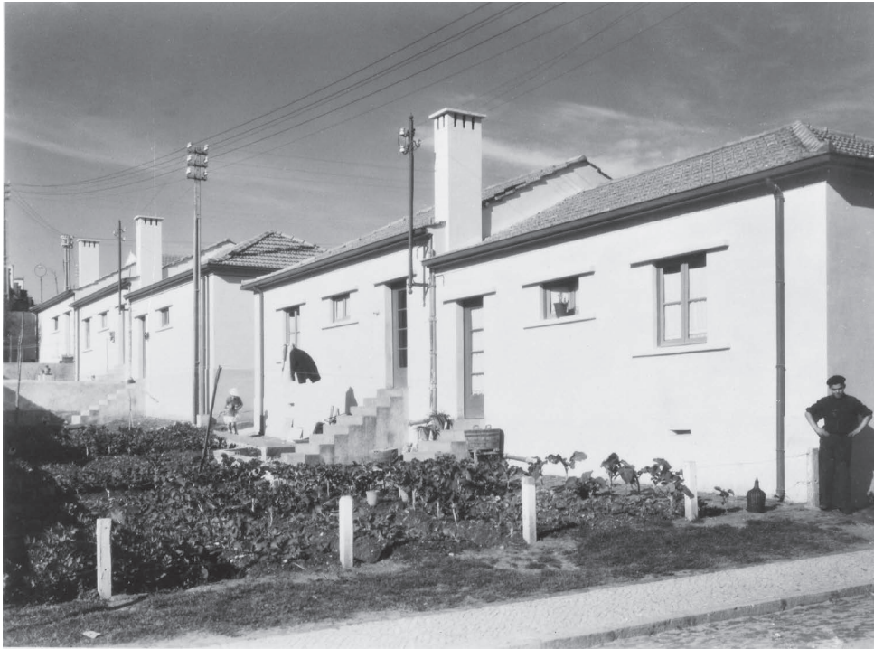
Fig. 2 Single-family houses in the Affordable Houses neighbourhood of Belém, Lisbon. Architect Raul Lino, 1933–1938. Source: Mário Novais Studio. Col. Mário Novais Studio [CFT003.023724.ic], Calouste Gulbenkian Foundation–Art Library and Archives.
