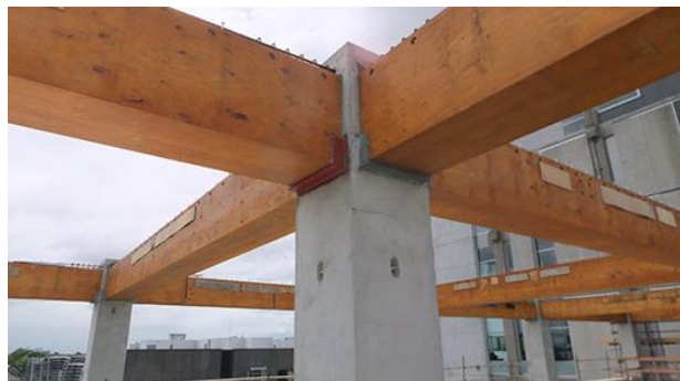
(b) hybrid joint: concrete-timber [30]
