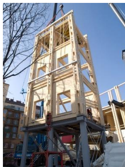
(a) hybrid construction [29]
