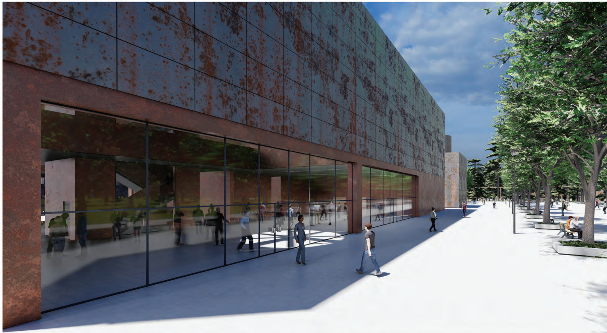
7 - External view of the Thermoelectric casting building
