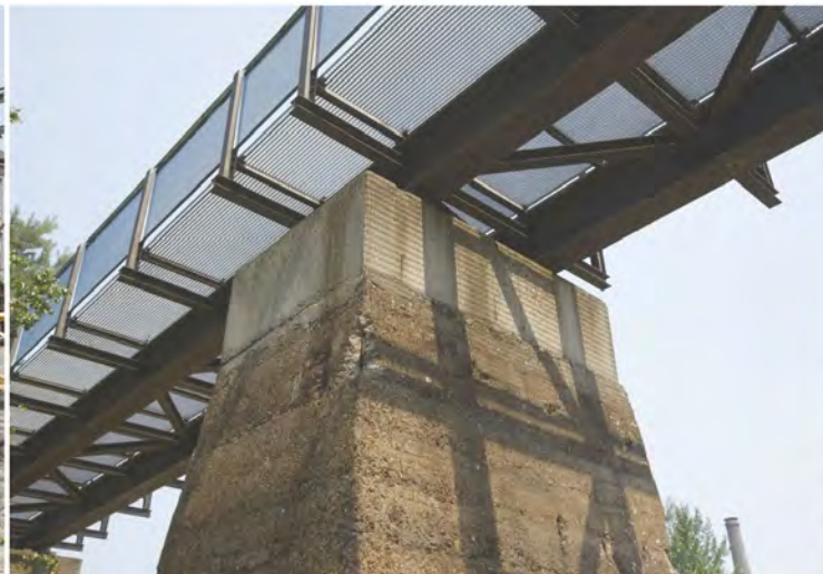
24- Reconstructed fallen railway bridge
