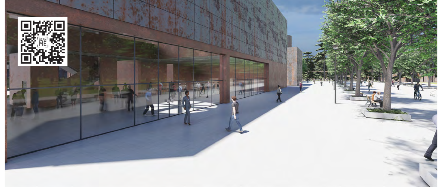
88 - External view of the thermoelectric cooling building (Scan QR for video)
