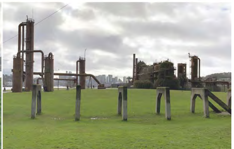
41 - Old concrete structures left untouched
