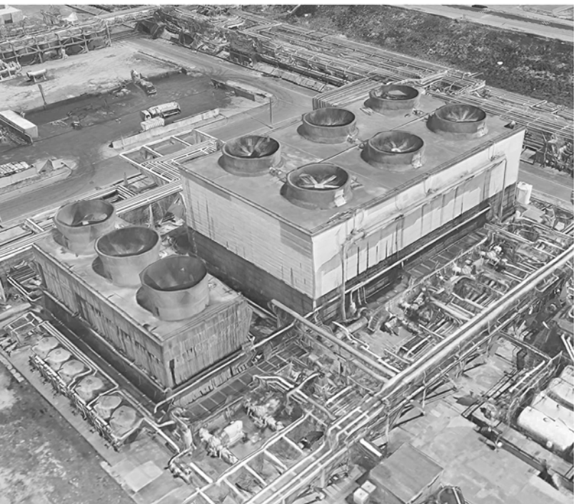
72 - Thermoelectric cooling buildings (southwest view)
