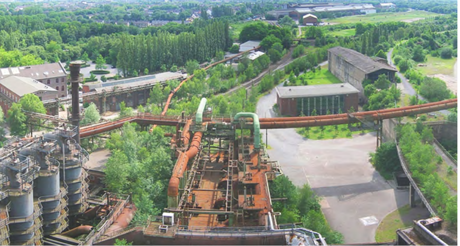
10 - Factory and infrastructure from above
