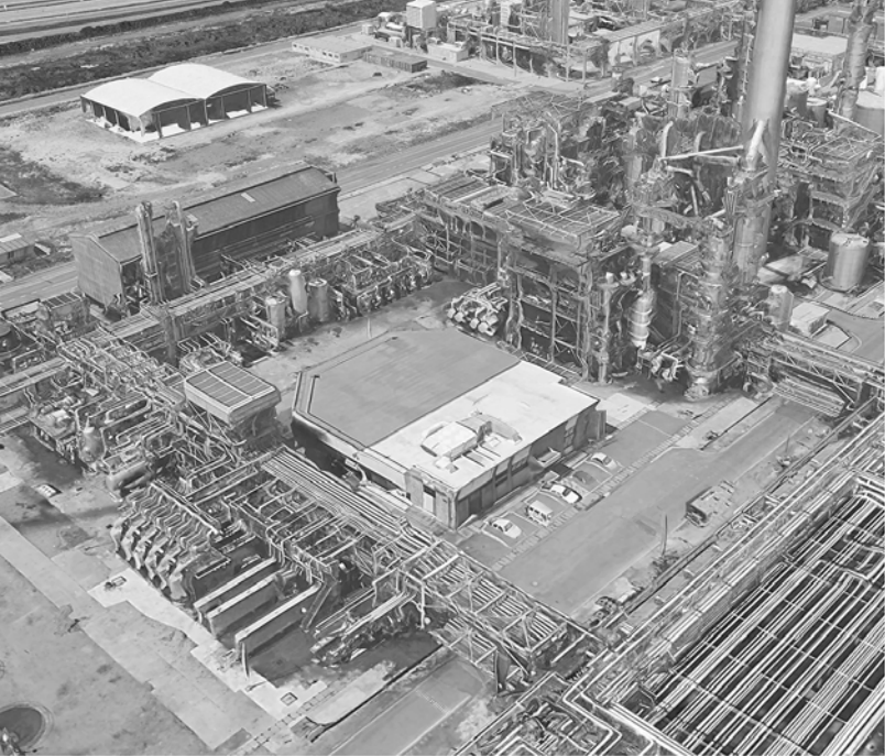
70 - Removed Office building
