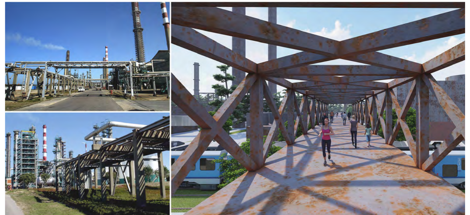
65 and 66 - Pipelines holding structure
