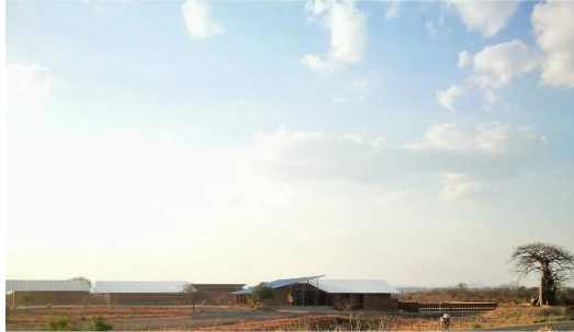
Figura 16: Benga Riverside Residential, vista exterior.
