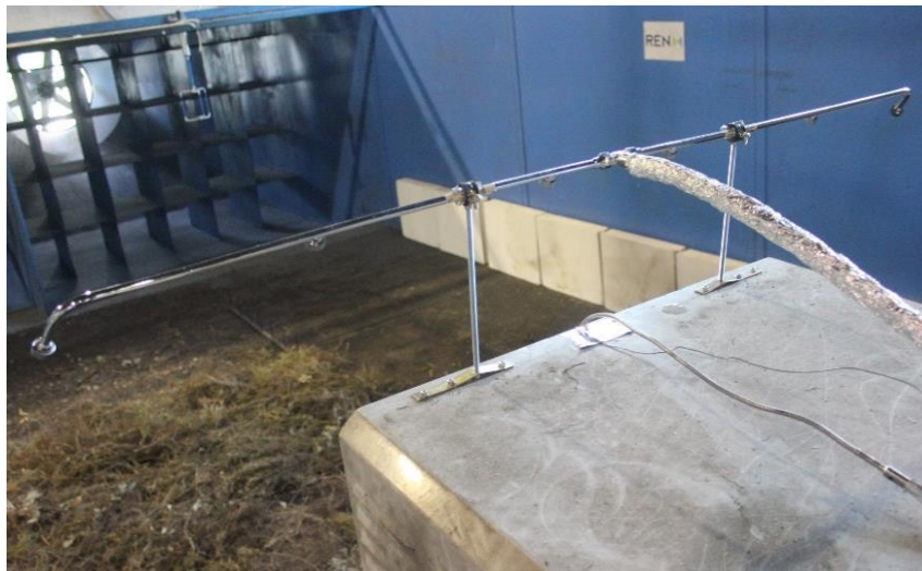
Figure 3.2 Position of the sprinklers at the top of the telecommunications cabinet.
