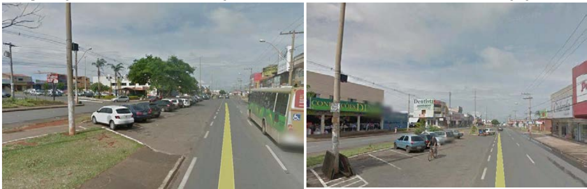
Fig. 1. (a) Initial section of a median parking area; (b) End section of a median parking area.
