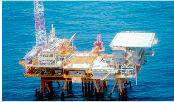
Fig. 2. General view of the Merluza-1 platform [8].
