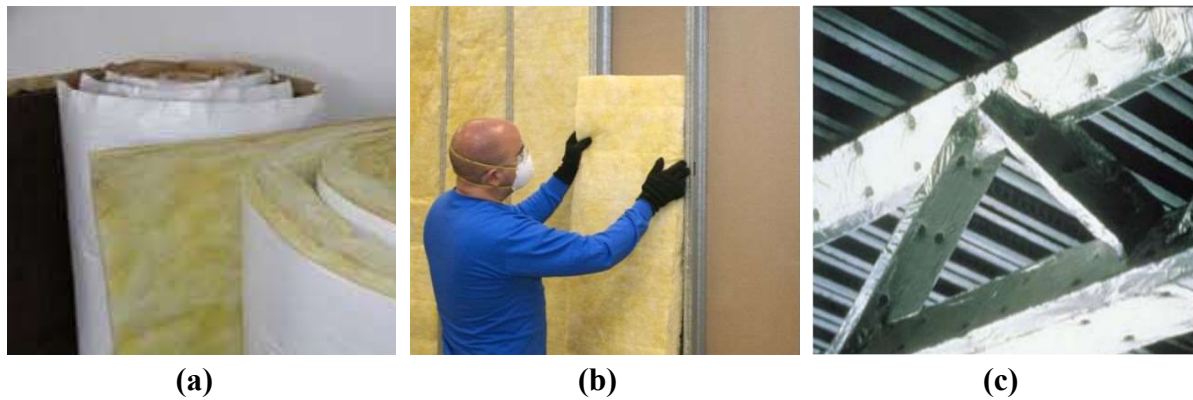
Figure 2.2 – Flexible blanket systems: rock wool (a), glass wool under installation procedure (b) and beams coated by the material (c) (from Ref. [45, 46 and 39], respectively).
