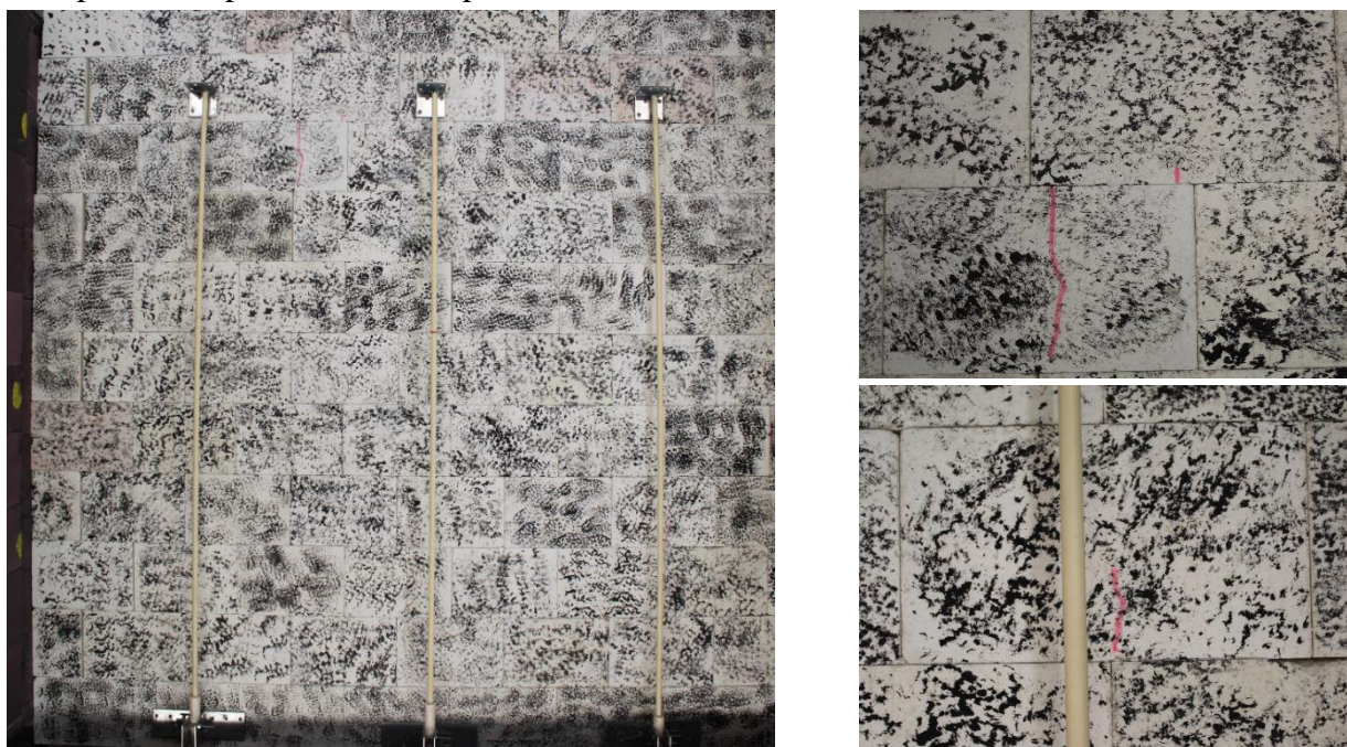
Figure 5-27 – Test series S06.AT.LBJ – Cracks observed in the specimen S06.AT.LBJ.01
