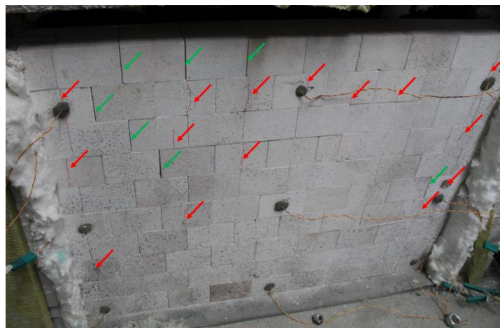
Figure 4-33 – Test series S04.HT.RTE – Failures in the wall: Vertical cracks in bricks and joints openings (S04.HT.RTE.02)
