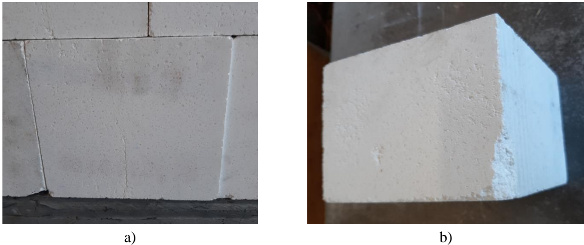
Figure 5-37 – Test series S08.AT.LBI – Cracks observed in the specimen: a) Cracks at cross joints; b) Crushing at head joint
