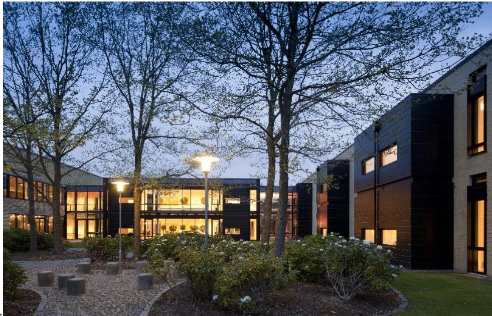
Figure 26 the external overview of building 210 (DTU 2003)
