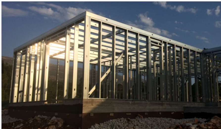
Figure 1 – LSF steel structure (Bloken, 2021a).
