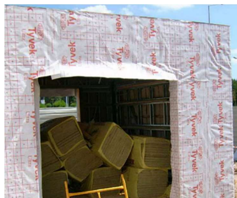
Figure 9 – Air tightness membrane (Soares et al. , 2017).
